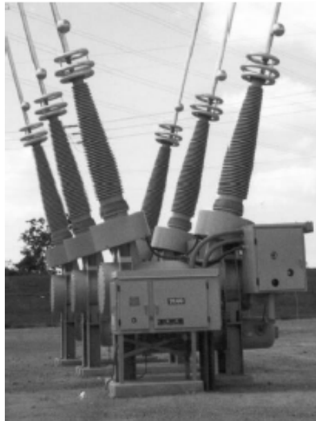
Fig. 13-25 SF_6 circuit breaker [5].
